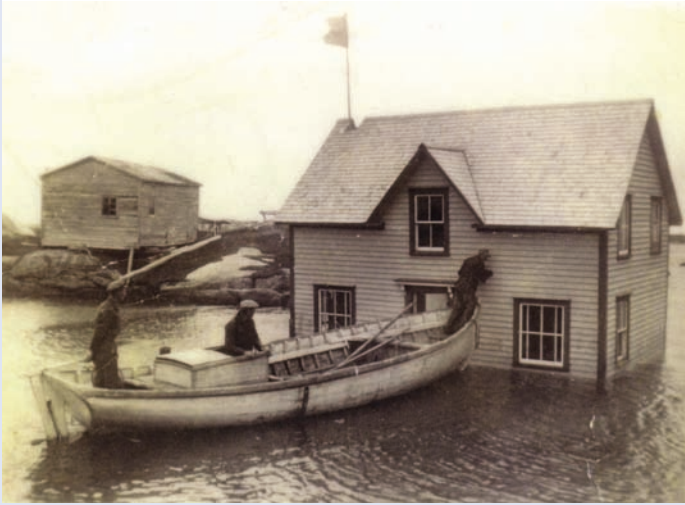
FIGURE 6–16 Resettlement continued in Newfoundland throughout the 1960s and into the 1970s. This house was towed across Inner Tickle of Newtown to its new location.
